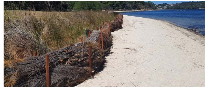
Soft bioengineering - brush walling
