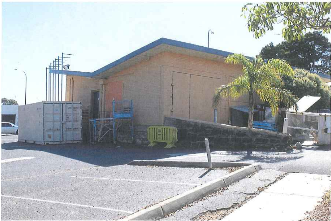
Captain Stirling drive through bottle shop south and east faces. Griffiths Architects April 2012
