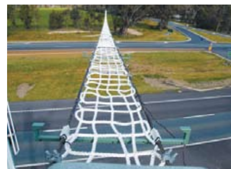
A rope bridge over the Hume Highway, Victoria, designed and installed by the Australian Research Centre for Urban Ecology (ACRUE, University of Melbourne) and VicRoads. Photo – Kylie Soanes (ACRUE) and Ross Meggs (Faunatech)
